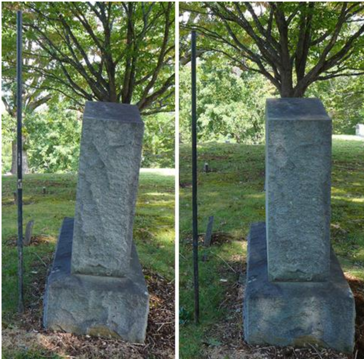
Roane family headstone; the bar is just under 6 ft long. I estimate that the stone, including several inches of base under the surface and concrete under that, weighs 3500 pounds.
