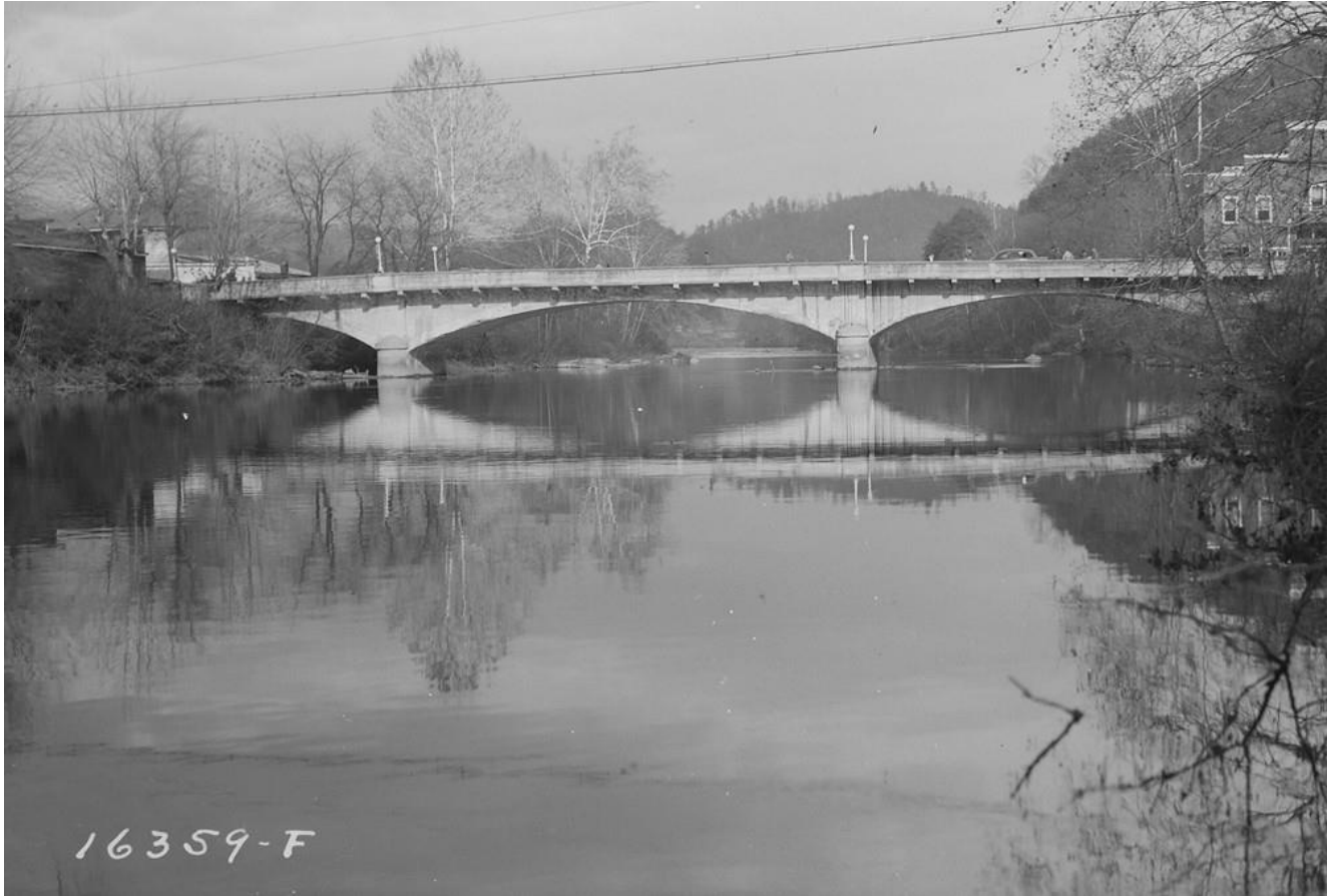
The Bryson City Bridge in 1942 (TVA photograph collection, National Archives, Morrow, GA)
