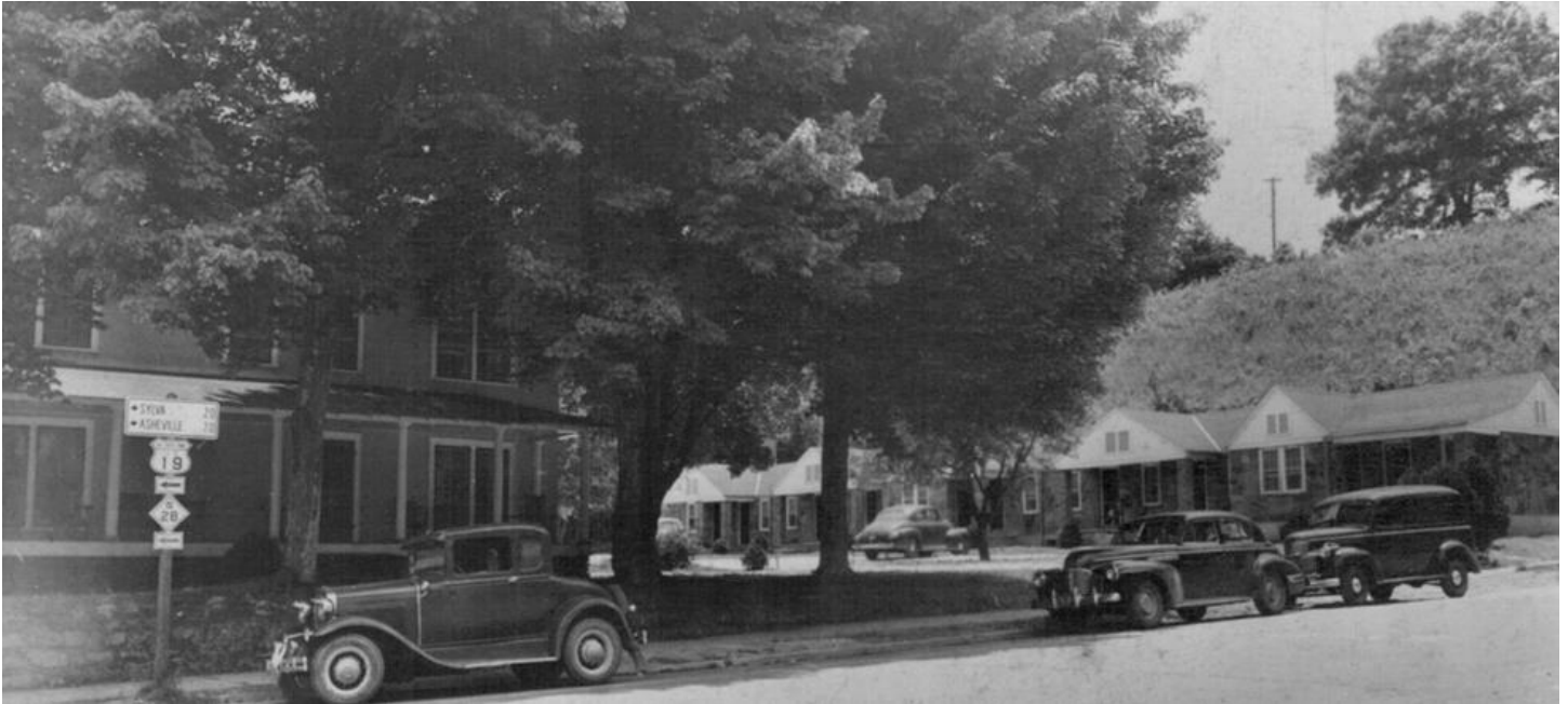
Figure 2. Jack and Sallie Keener Franklin home and Rhododendron Motor Court. Source: Jim Casada
