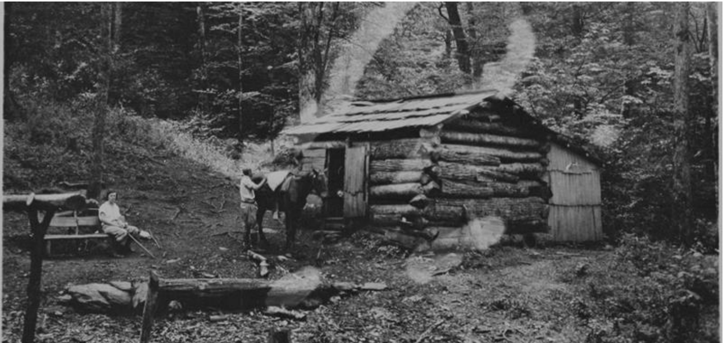
Figure 18. Moore Spring cabin, near Gregory Bald. Source: Open Parks Network
