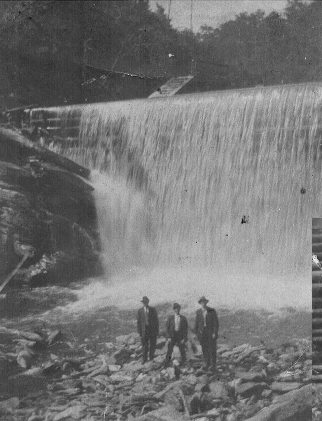
Deep Creek dam and powerhouse; photos courtesy of Jim Estes
